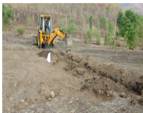
The soil dug out, before replantation.
